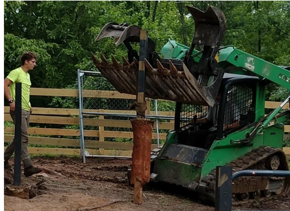
2020 Paddock Fence Repair Project
